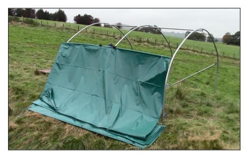
4 Centralise the PVC cover in length and width and pull the cover over the end arches. Temporarily tie off the ropes to the "side" ridge tubes.
